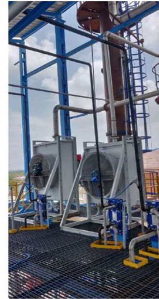
CEES Air cooled Alcohol vapor condenser
